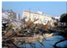
Loma Prieta Earthquake
